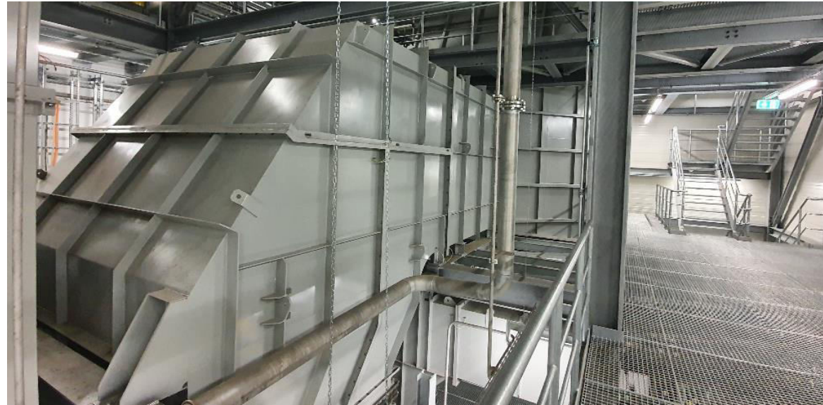
Filter House Sliding by Oil Hydraulic Skidding System & Duct Installation
