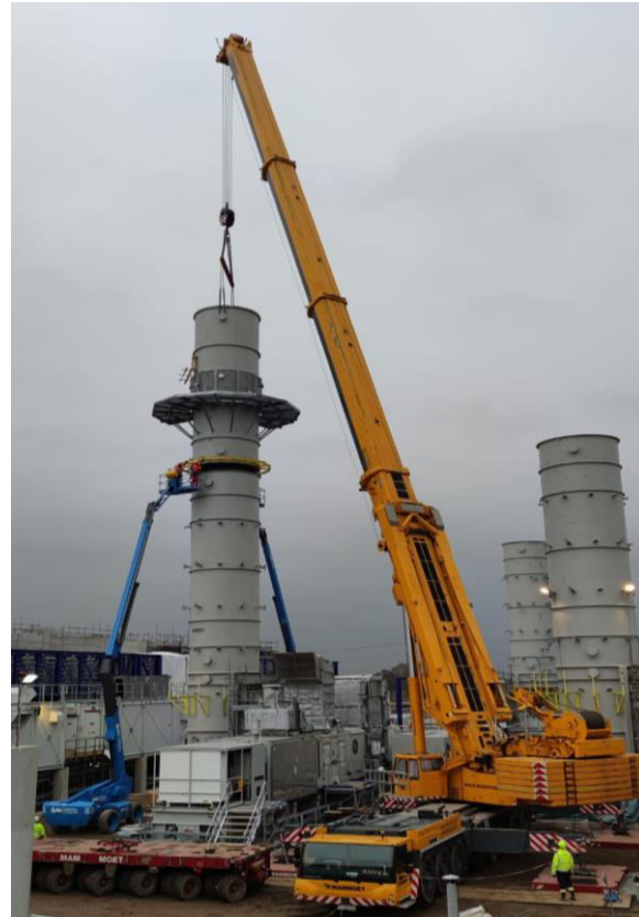
STACK ERECTION
