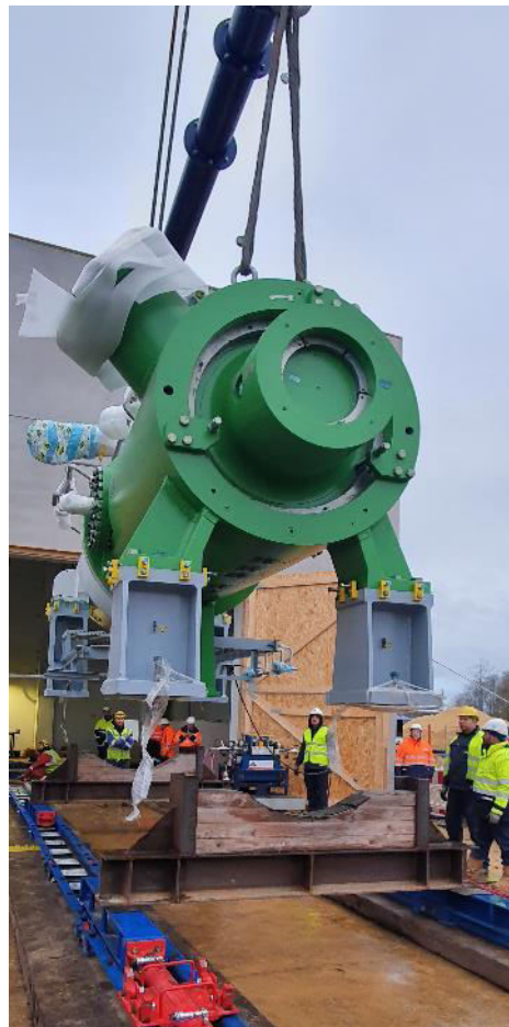
ICL COMPRESSOR LIFTING
