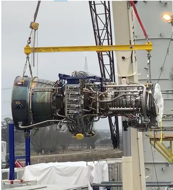
ENGINE LIFTING OPERATIONS
