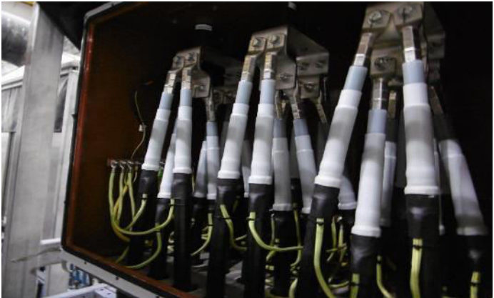
MV termination – Step Up Trasformer
