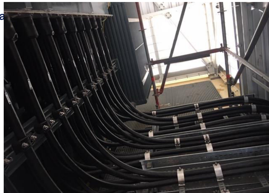
MEDIUM VOLTAGE CABLES LAYING
