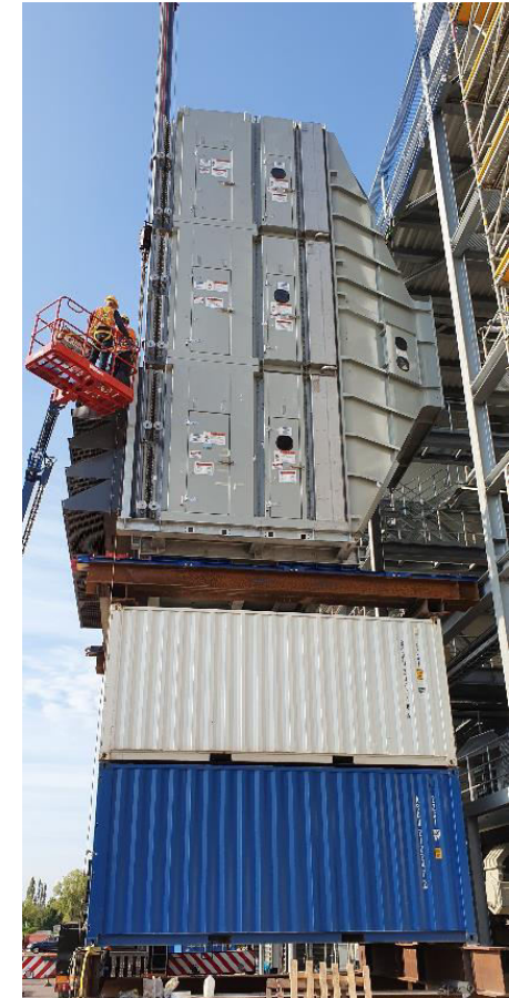
Filter House Sliding by Oil Hydraulic Skidding System & Duct Installation
