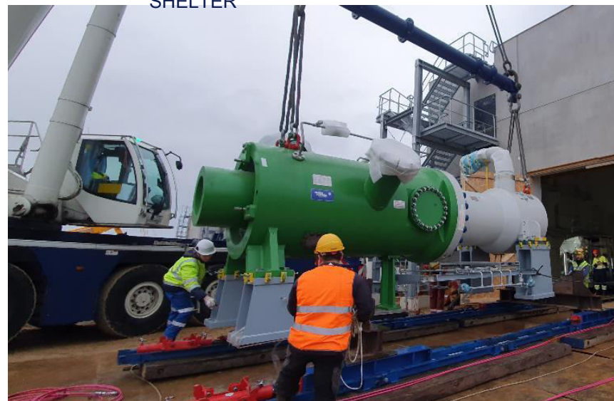
ICL COMPRESSOR SLIDING SYSTEM
